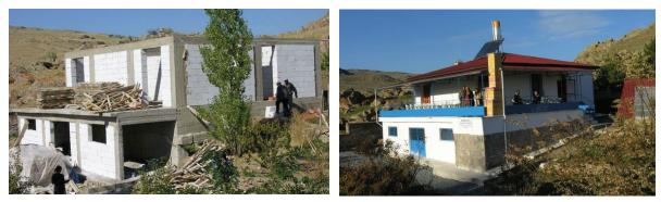
Figure 6. The Erdoğan Akdağ Center was built with a concrete frame and AAC blocks infill.
