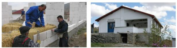
Figure 7. A hybrid construction technique of AAC blocks and straw bales was used for the Kerkenes Stone Conservation Building.
