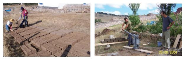
Figure 9. Traditional sun dried mudbricks (left) and pressed bricks (right) were produced at Kerkenes and used for small projects designed by students.
