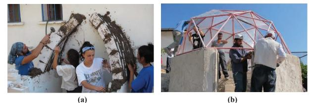
Figure 11. (a) A small Nubian vault built with AAC blocks and (b) construction of a geodesic dome during Hands-on course at Kerkenes.
