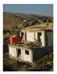
Figure 5 : Building with Aerated Concrete and reinforced concrete frame
