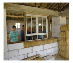
Fig 1. A window is being installed in the underconstruction hybrid wall of the Strawbale-cum-AAC building.
