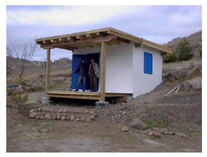
Figure 14. The mudbrick walls of the unit structure have stone foundations. The flat mud roof, with its timber ceiling and rafters, is supported by beams and posts built into the walls so as to make the structure earthquake resistant.
